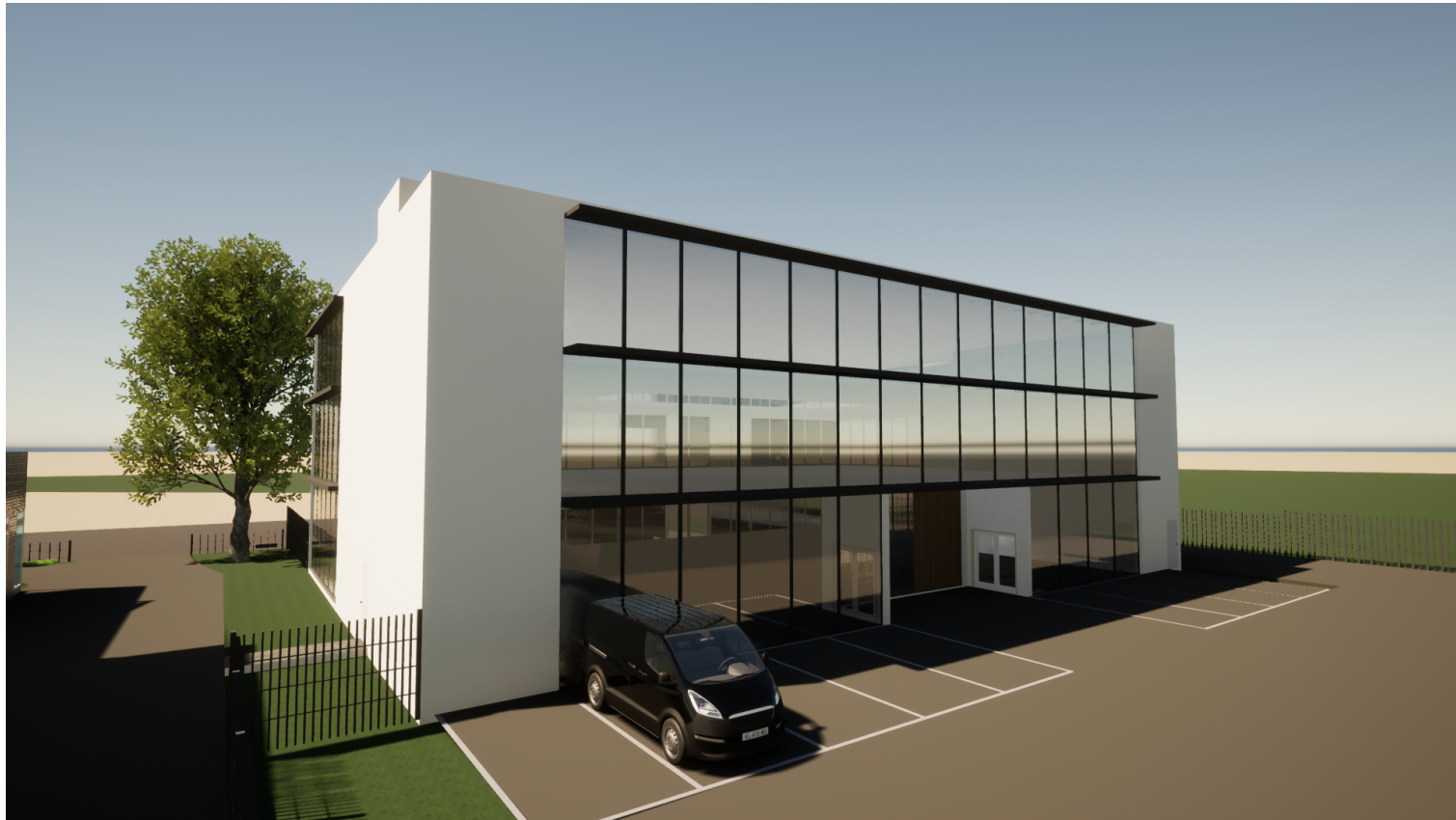
NORTH WEST (FROM CARPARK)
